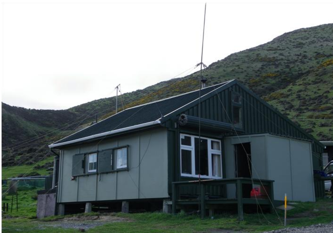
Antenna at front is a WW2 vertical - ZC-1 I think! Main antennas on pole erected at the back of shack
