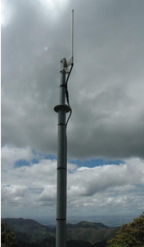
23cm antenna on old metal pole
