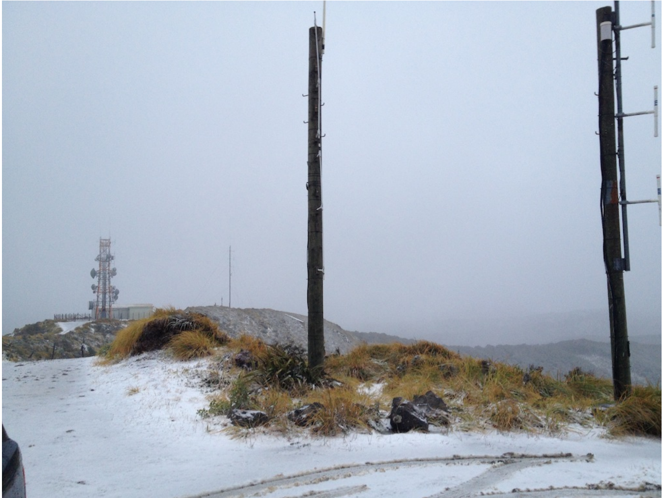
Snow at Mt Climie on Sunday 14 July 2013 – looking south at Telecom Tower
