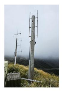
This will allow us to remove the old 10GHz beacon pole as it is now beyond its safe usable life. The battery box seen in the foreground will enable us to install more batteries so the 6m 395 repeater can have battery backup and provide 12v power for the wi-fi link and SDR.
