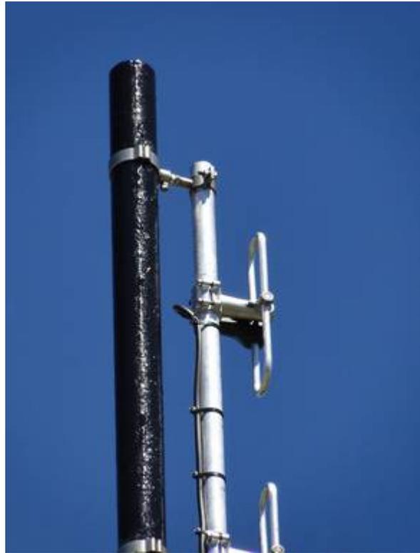
The following pictures show the encapsulated phasing harness and a close up of a single dipole construction.
