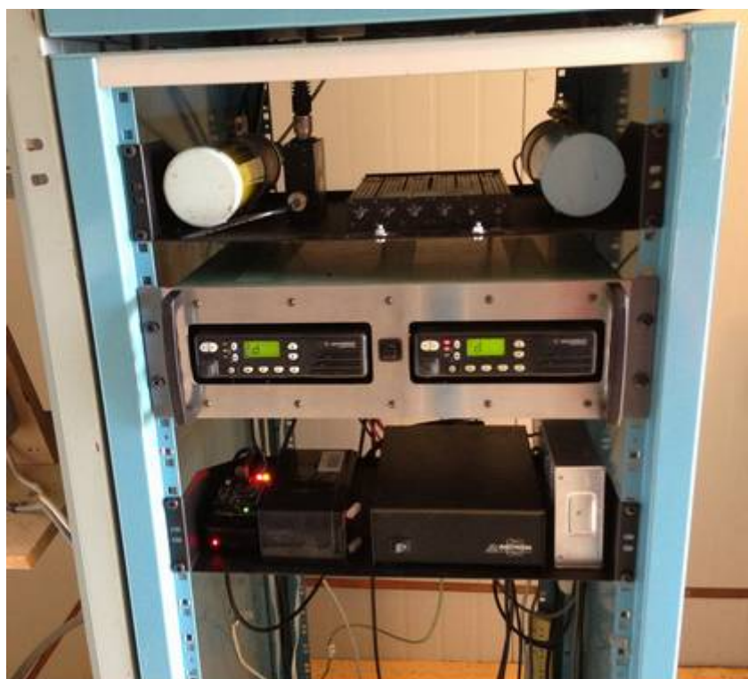
ZL2HBD UHF Installation Mt Threave.
