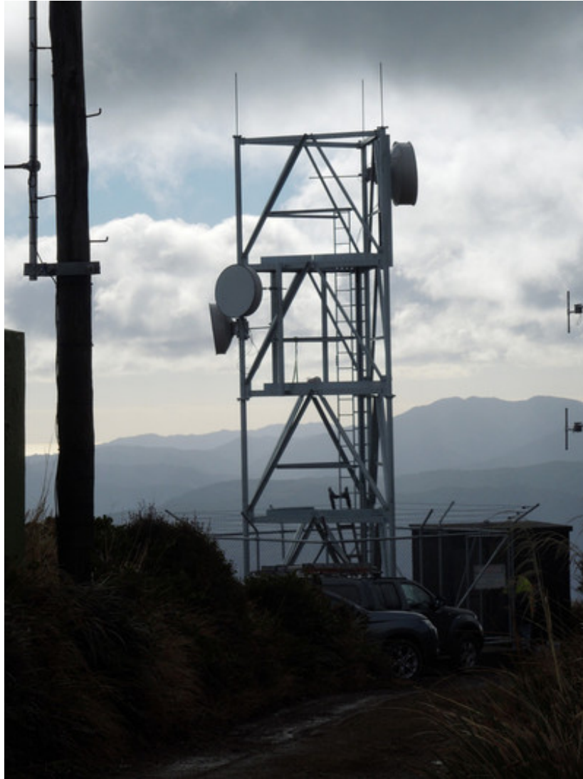
New north tower used by waterboard
