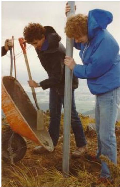
Upon completion of the four foot deep hole, Richard ZL2UGC holds the bottom section of the mast while Michael ZL2TDT pours the concrete.
