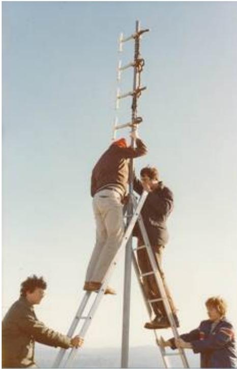
Paul ZL2UGR and John ZL2TWS bolt the two flanges together leaving a free standing antenna system. ZL2TDT (ZL2BPL) and ZL2UGC give some support.
