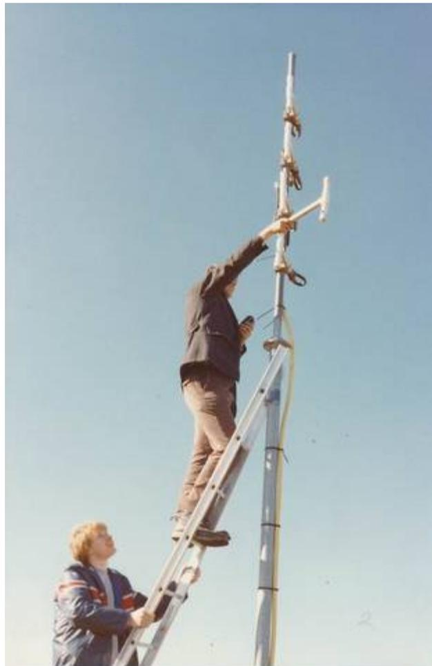
The completed installation. Power was measured at dipoles as 15 watts feeder loss 0.54db. First contacts Jeff ZL2CW and Gretta ZL2AGS. Then John ZL2TRV (ZL4RF) spoke to Ralph ZL1TBG in Walkworth north of Auckland. The machine worked well.
